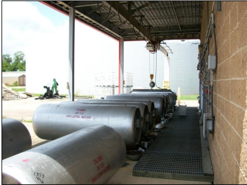
Figure 1-2 Chlorine Cylinders at BWA WTP
